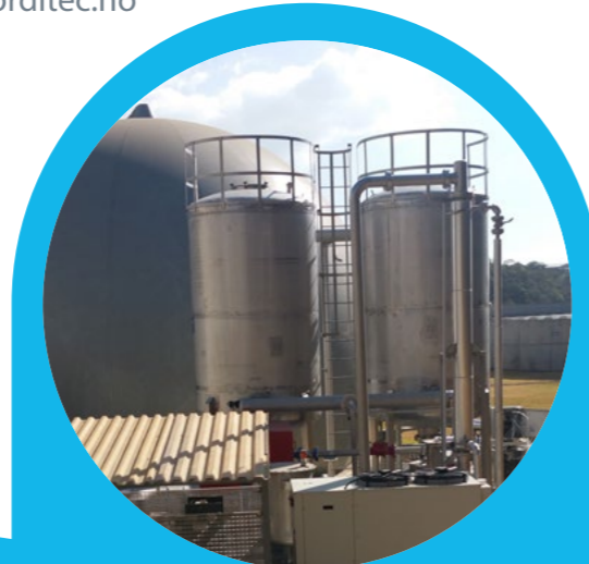
Overview of the plant
