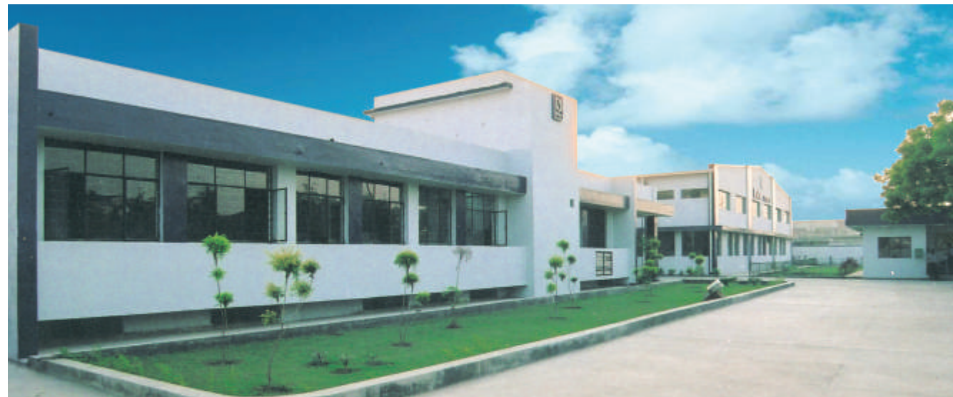
Roto's Manufacturing Plant
