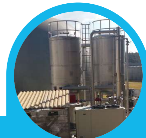
Biogas cleaning
