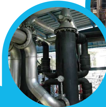
Biogas Dryer
