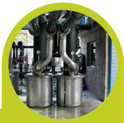
Inside water vapor removal
