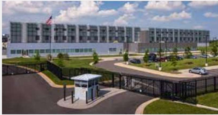
Amazon Data Centre, USA (Northern Virginia)
