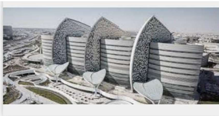
Data Centre In SMRC, Qatar
